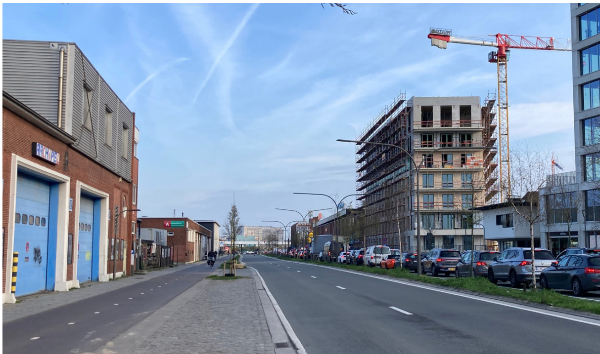
Figure 3. Archipel occupies the building on the left side, with across the street the redevelopment site of the former slaughterhouse (Authors' picture, 2026).
