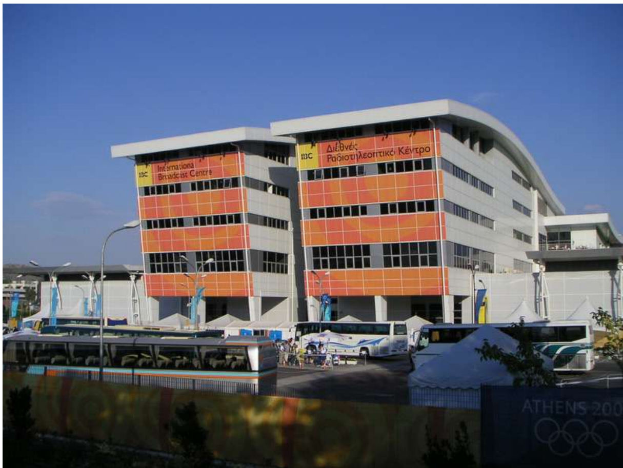
Figure 5: International Broadcast Centre. Source: https://digitalvinfo.gr/arthrografia/technologia/ibc-international-broadcast-center/
