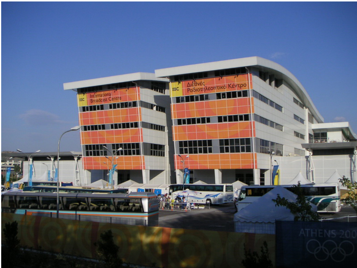
Figure 5: International Broadcast Centre. Source: https://digitalvinfo.gr/arthrografia/technologia/ibc-international-broadcast-center/
