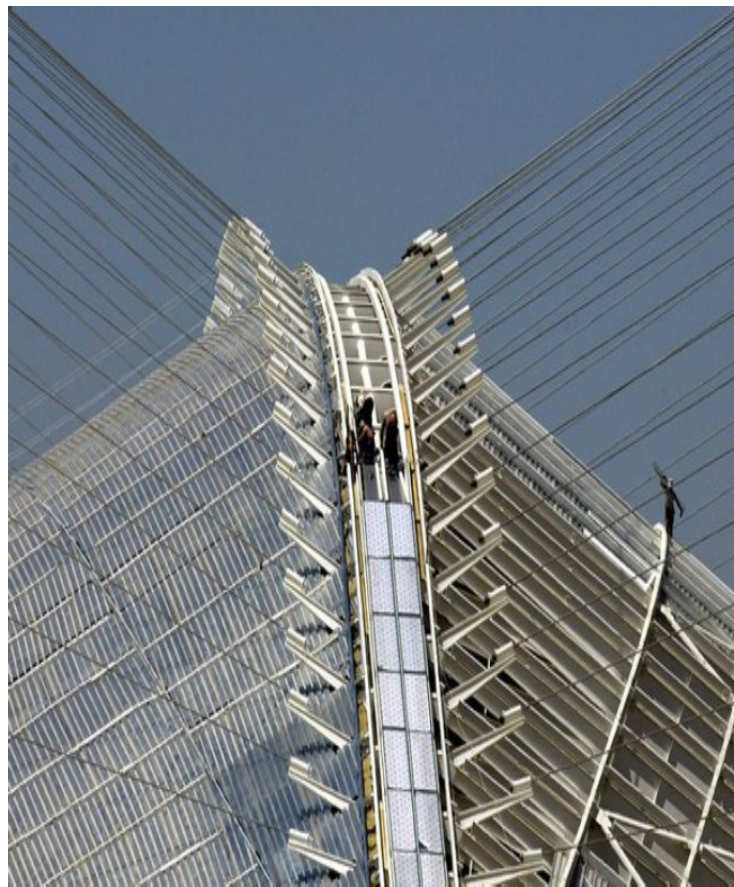
Figure 3: Athens Olympic Stadium. Constructions in the steel dome after its closure in September 2023. Source: Monocle Minute , 04/10/2023
