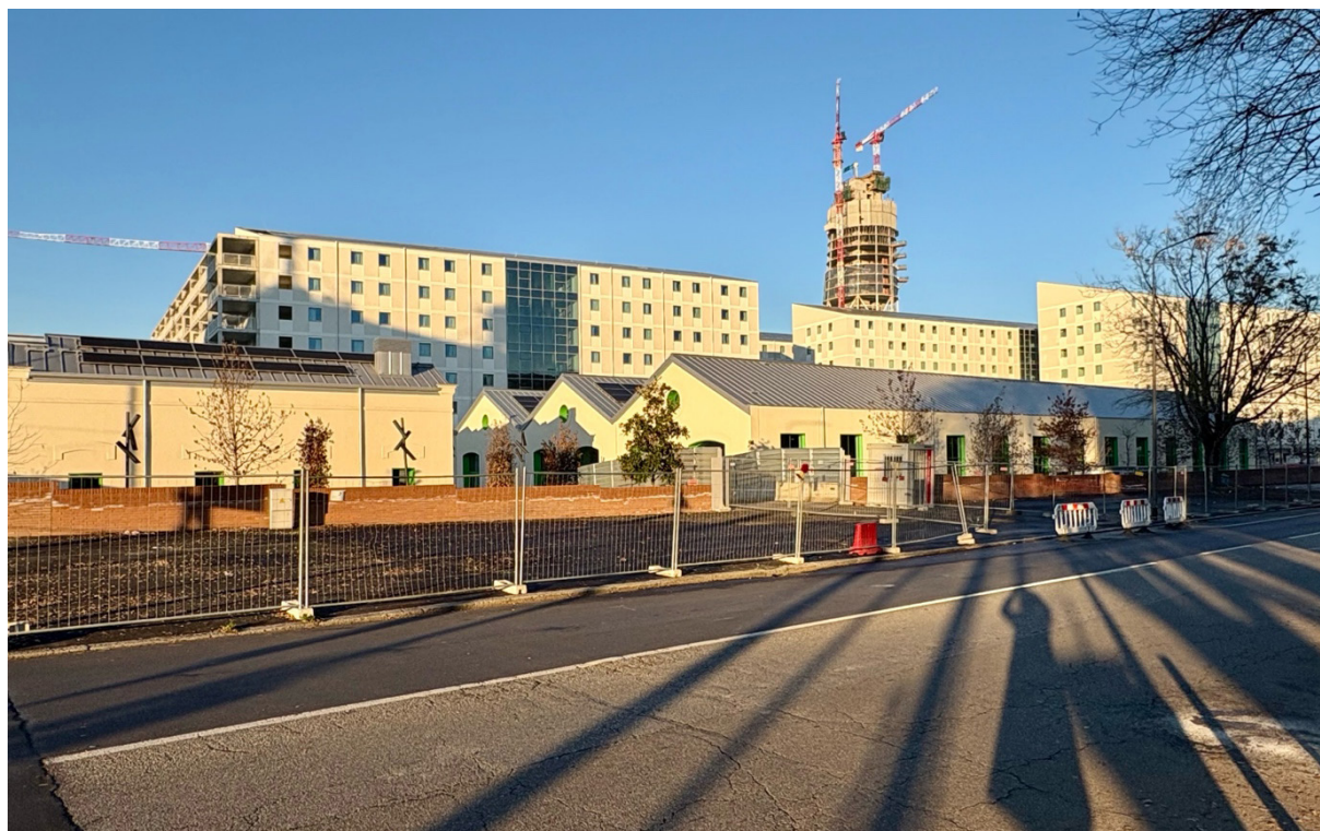
Fig. 4. The construction site of the Athletes' Village at Porta Romana in December 2025, two months prior to the opening of the Games. Source: Authors
